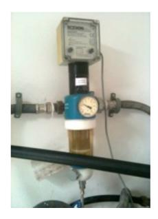
d. Check if the water pump for domestic water is working correctly building periodically sufficient pressure of (max 3.5 bar).
