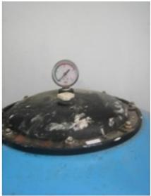
If is to high make a BACKWASH procedure. ( see instructions Sand filter cleaning)
